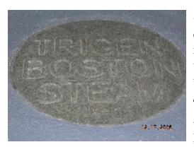
**Customer Benefits:** The FRP composite manhole cover surface is non-conductive. In service, the manhole covers must handle 400 F temperature underneath the lids while maintaining a surface temperature of under 170 F.
